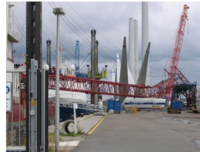
A crane collapsed in the marshalling harbor
